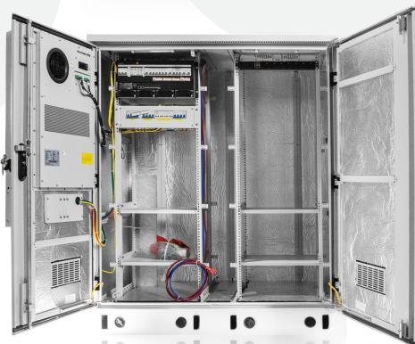
A freestanding cabinet with a height of 32U, designed for outdoor use. Constructed from 1.5 mm thick 201 stainless steel, providing high strength and resistance to harsh environmental conditions. The cabinet features 20 mm polyurethane insulation and automatic temperature control - if the internal temperature exceeds 35 °C, the air conditioner is activated automatically.
